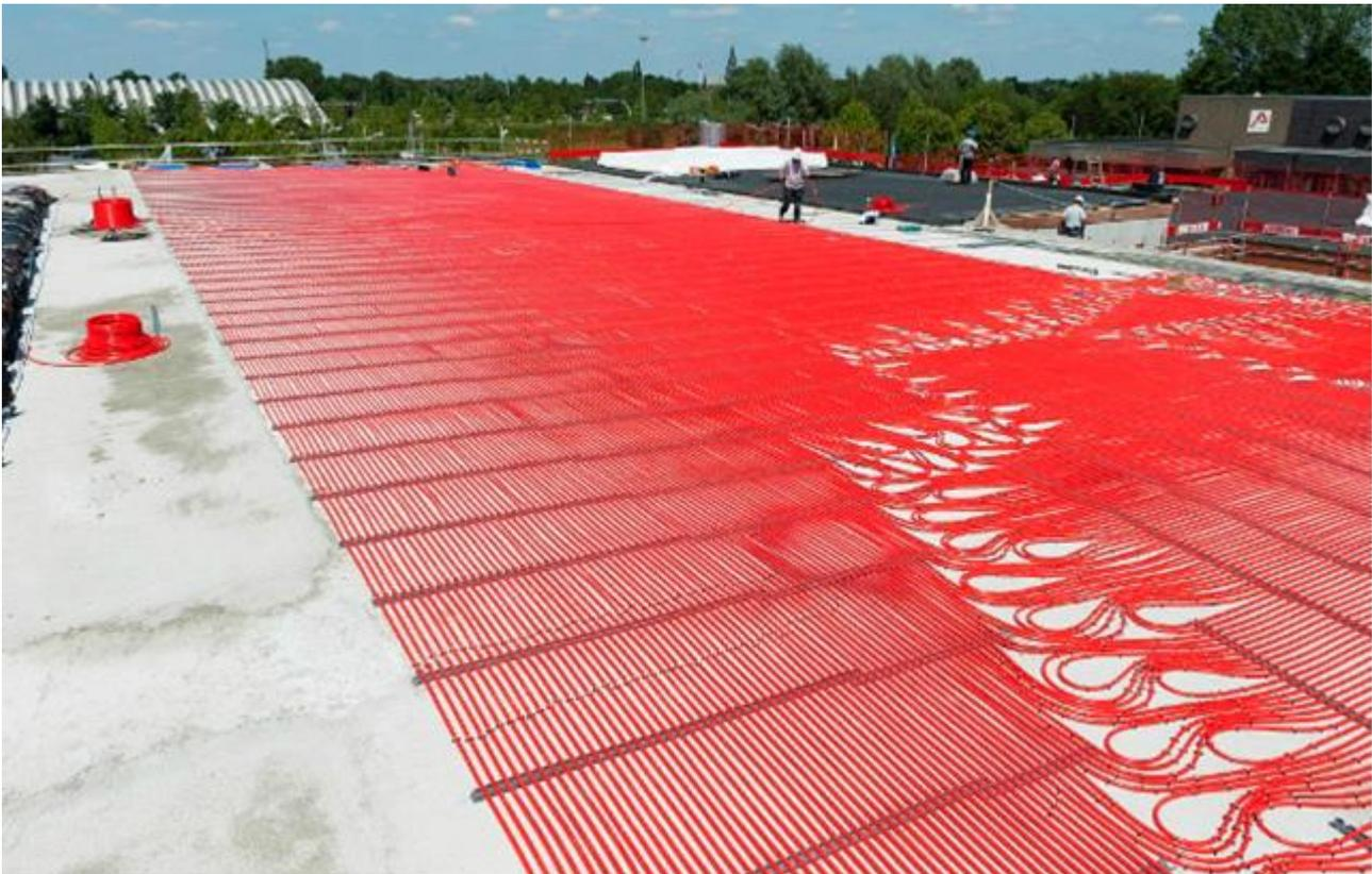
Fig.2 Build-up of the energy roof
